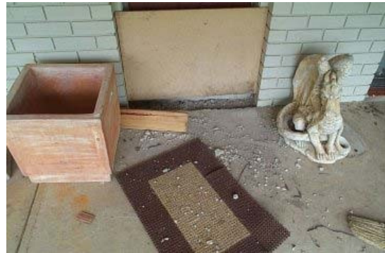
This door was boarded up which was no obstacle to a determined wombat. You can see that the wombat dug up the concrete in an attempt to get inside (83)
