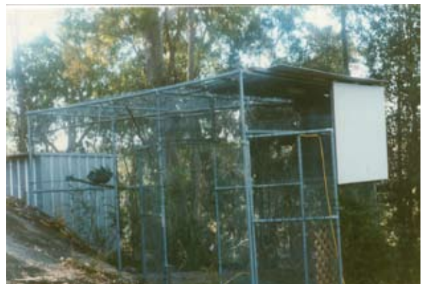
Outside aviary (purpose built) recommended size 2400mm high by 2400 wide by 4800 deep
